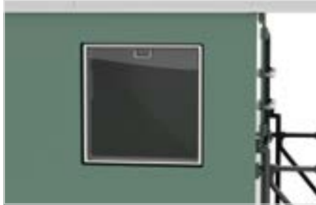
Perfectly-installed full-drop windows
